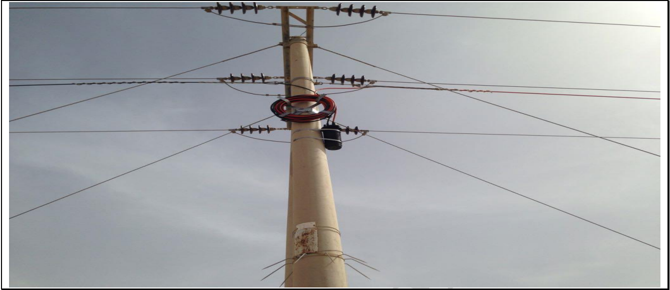
Cross - Aerial Cable Storage Configuration With Cross-bar
